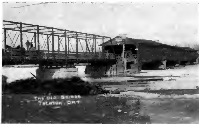
The Old Bridge at Trenton, Ont.
